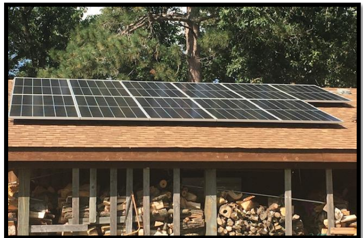
New solar panels installed at Lin & Joel Ward's place.
