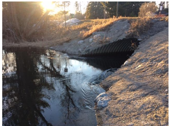
Water through the culvert-04-09-19 photo by Joel Ward
